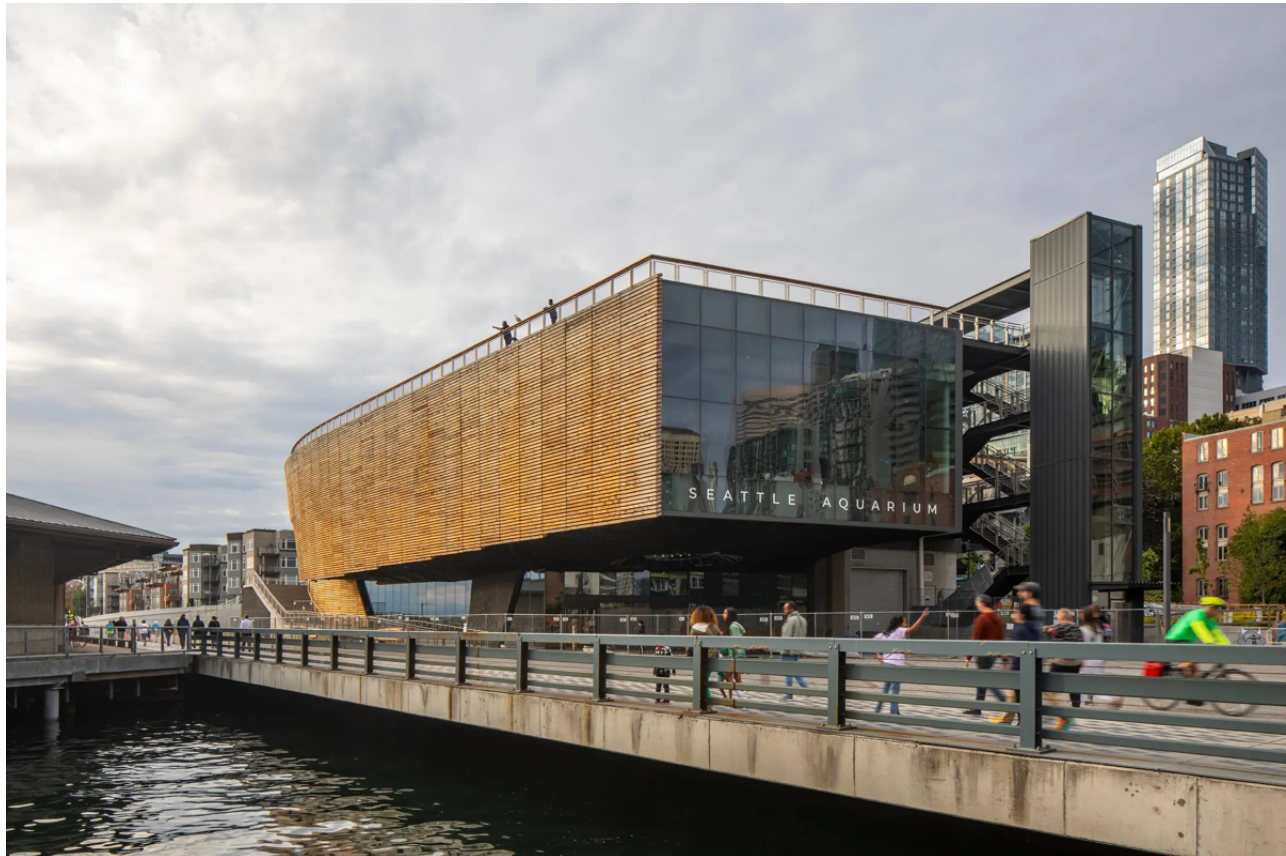
The Seattle Aquarium's new Ocean Pavilion and public plaza. The skin and facade of the building is Alaskan yellow cedar, metal panels and glass. Lara Swimmer/ESTO
